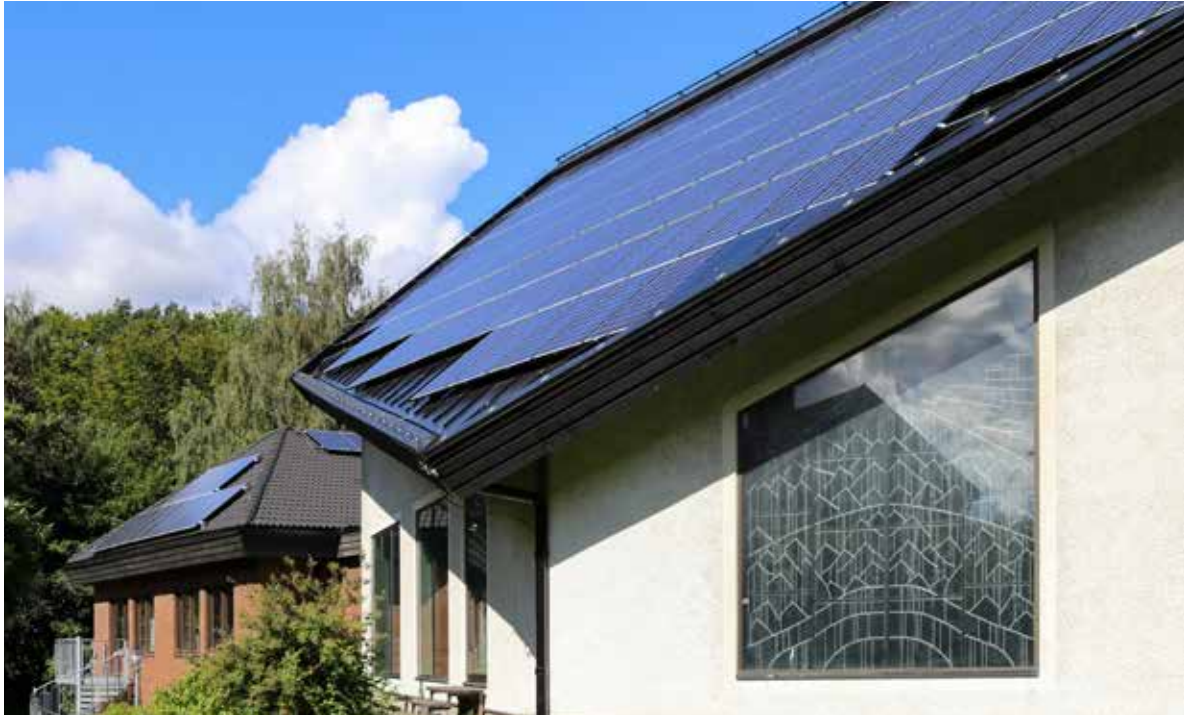
The church in Vargön in the Parish of Western Tunhem, power from above. Their electricity and heating have come from solar panels on the roof for the past three years.
