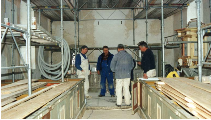
Håkantorps kyrka under renovering.
