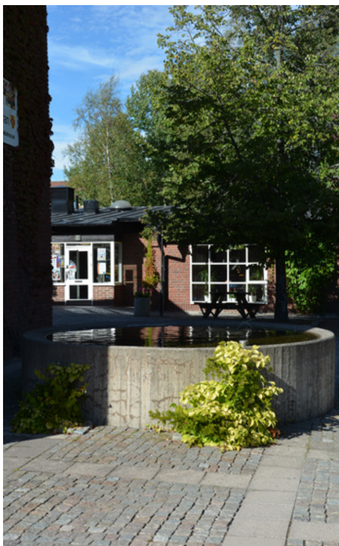
Springbrunn gjuten i betong. Vlm_modkaEK-2874.
