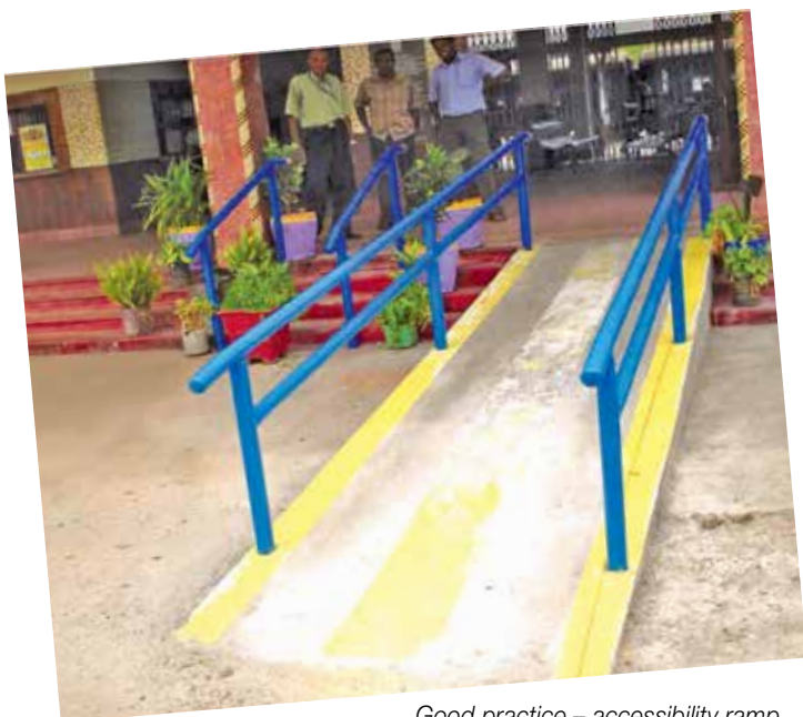
Good practice – accessibility ramp
