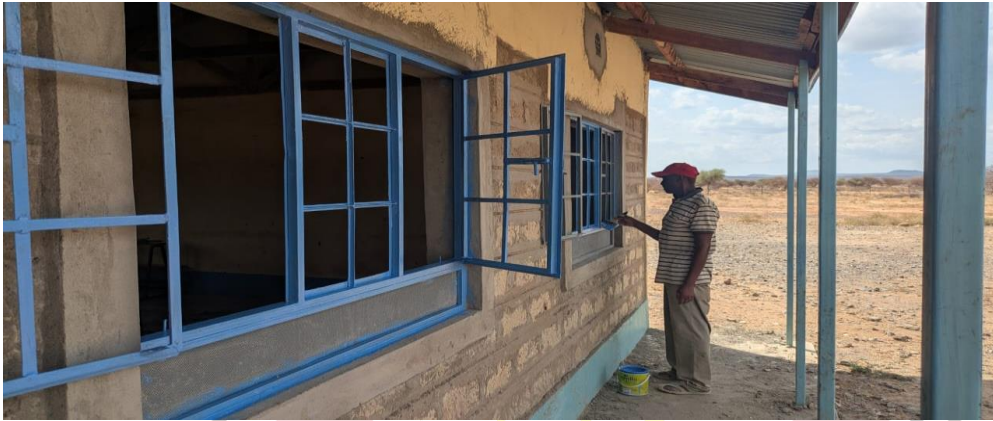
An old classroom being repaired.
